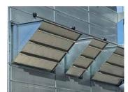
6 The pressure relief surfaces increase safety in the event of an explosion. An opti-
